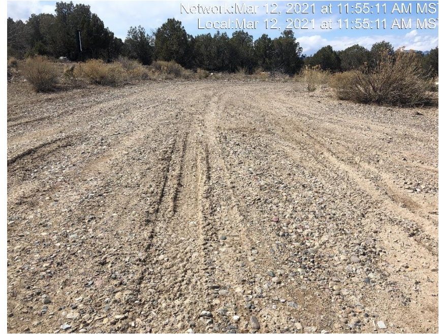
Photo #3132 No tracking control at entrance to location.
