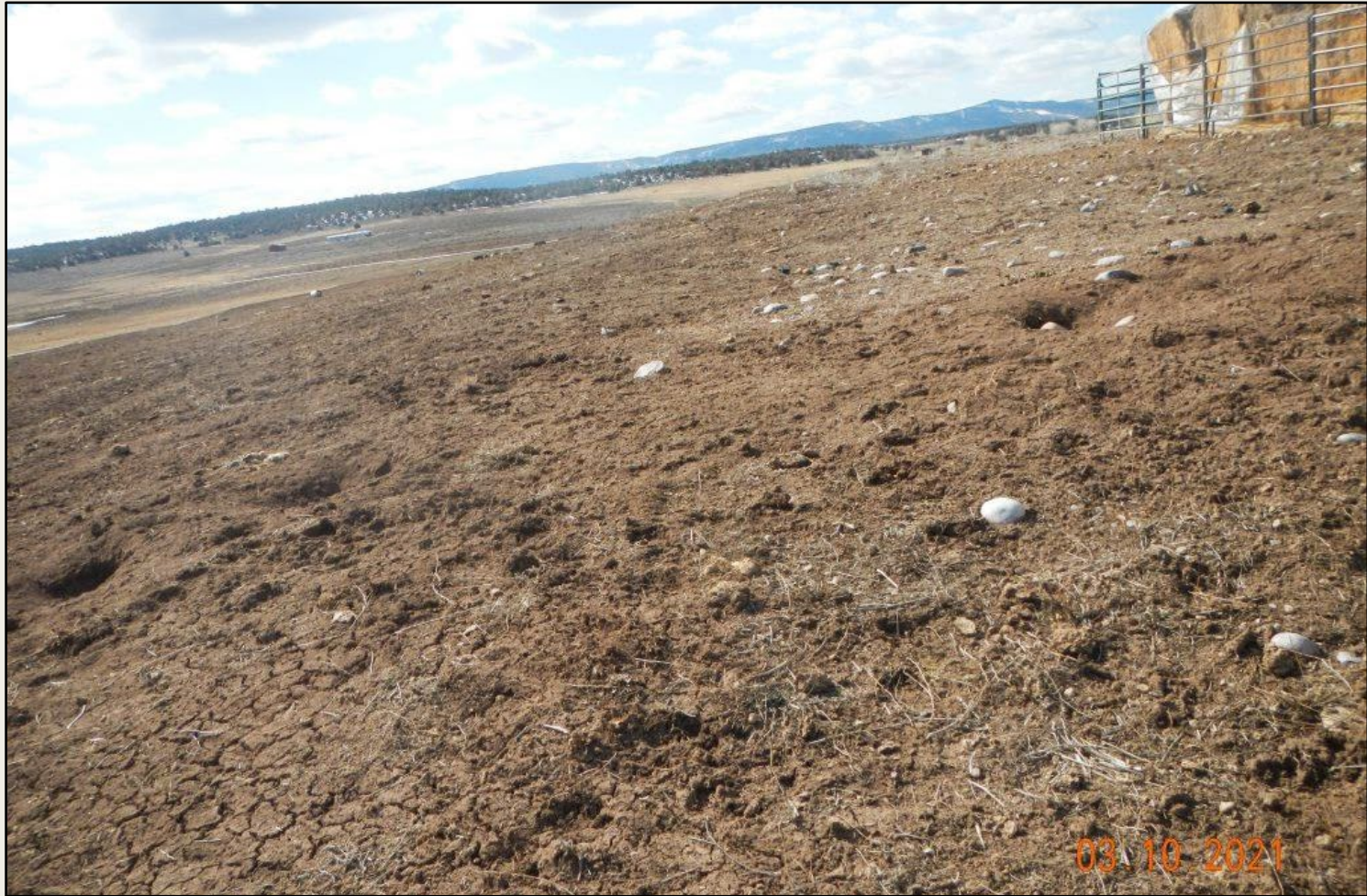
Photo 2. View of the eastern fill slope from the northeastern corner facing southward. Perennial vegetation observed is in a grazed condition and needs to be monitored during the active growing season to ensure site stabilization.
