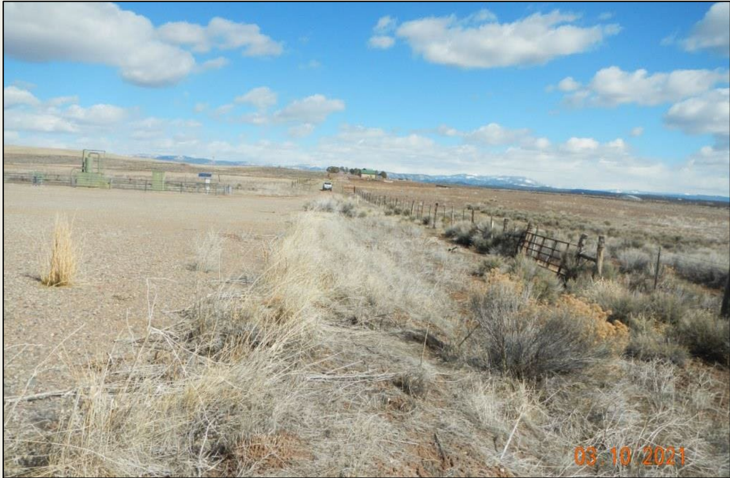
Photo 2. View of the eastern fill slope from the southeastern corner facing northward. Revegetation is largely dormant, but comprised of western wheatgrass, rubber rabbitbrush, and crested wheatgrass.
