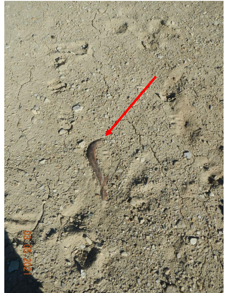
Photo#3: Anchor run over and buried in pad surface.
