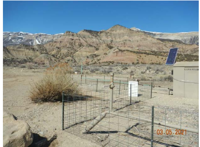
Photo#3: View over equipment to Interim.
