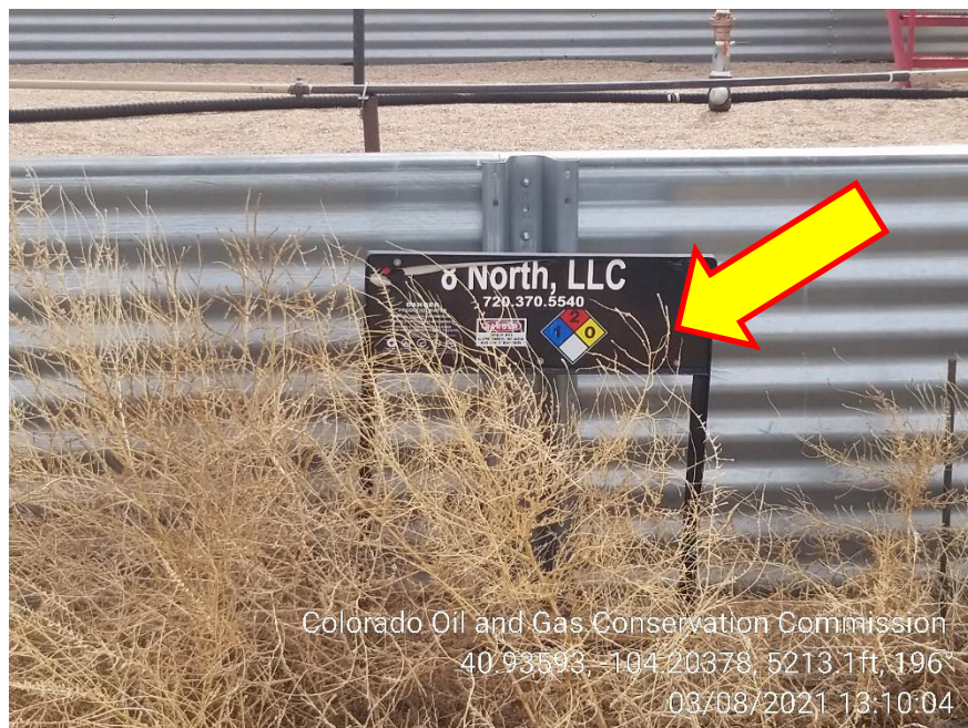
Photo 3 – Missing Capacity Label, Weeds
