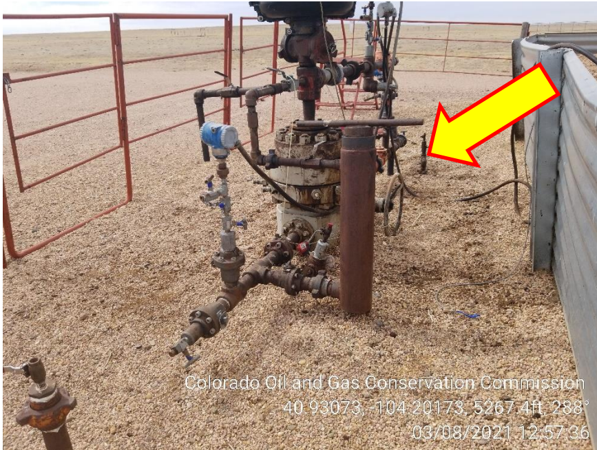
Photo 3 – Unmarked Riser
