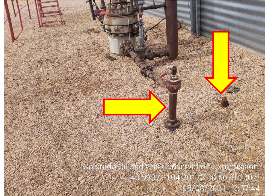
Photo 4 – Unmarked Risers
