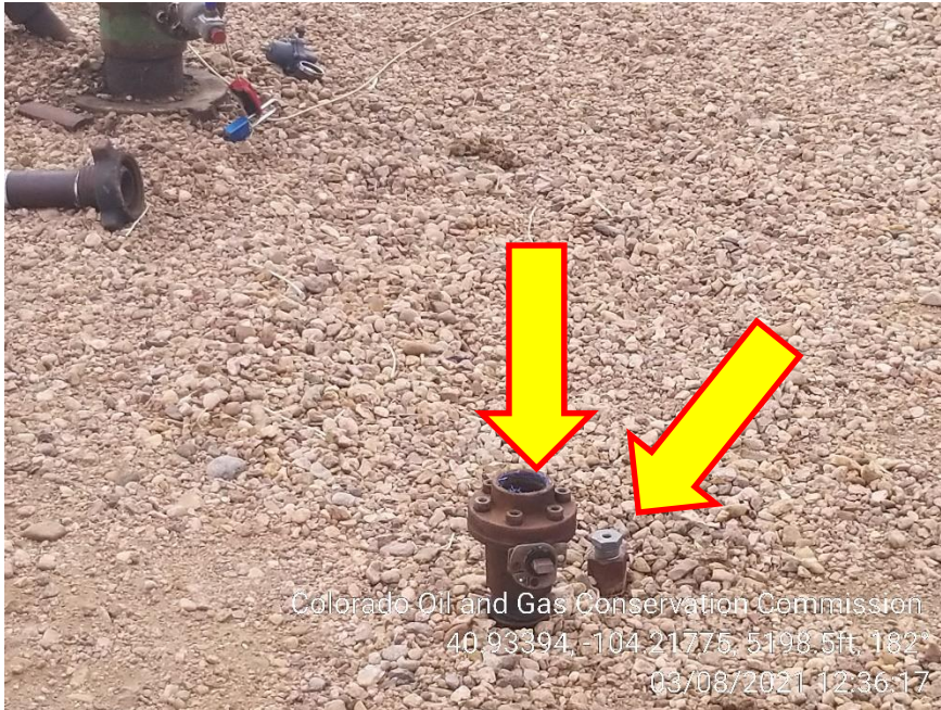
Photo 5 – Unmarked Risers
