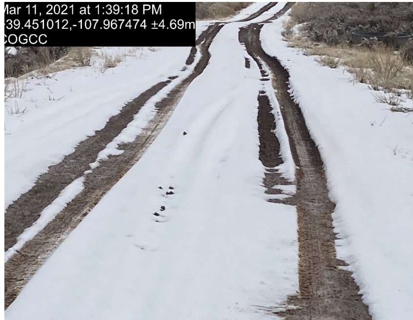
Location entrance/lack of stabilization/compaction
