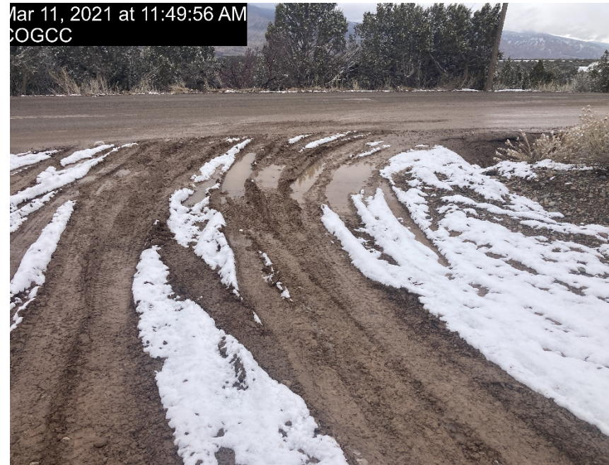
Heavy Tracking onto county road from lease road is occurring. No tracking BMP are present at the time of inspection. Lack of stabilization/compaction.
