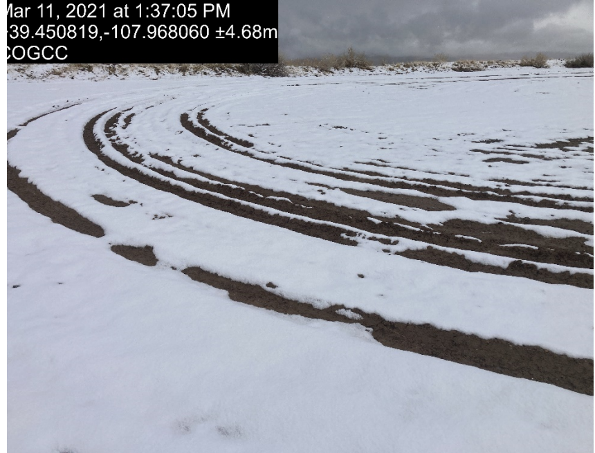
Lack of stabilization/compaction on location
