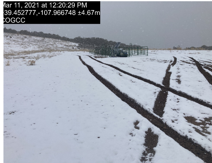
Location around well heads still shows signs of lack of stabilization/compaction
