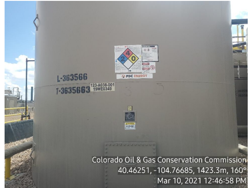
Photo 4: No BBLS displayed on crude oil tank.
