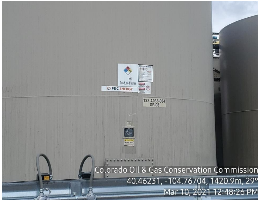
Photo 5: No BBLs installed on H2O tank
