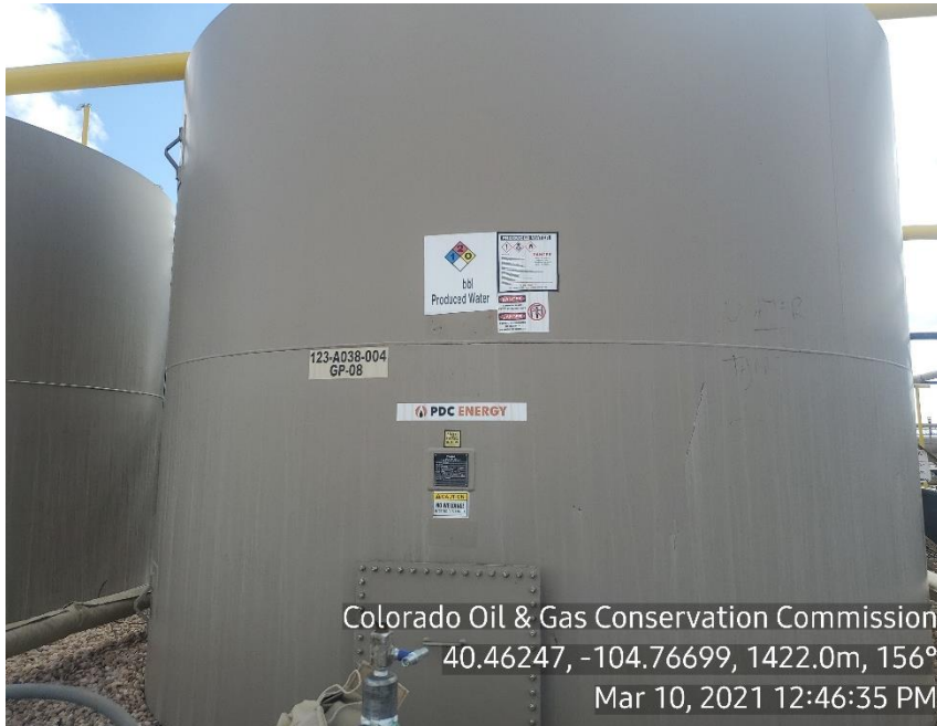
Photo 3: No BBLS displayed on H2O tank
