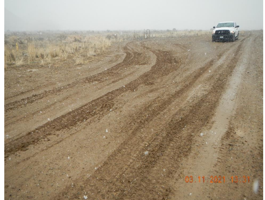
Access road and location lack stabilization.
