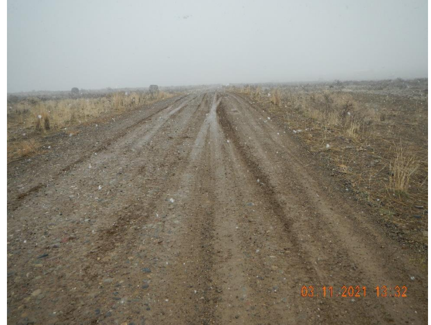
Access road headed northeast lacks stabilization.
