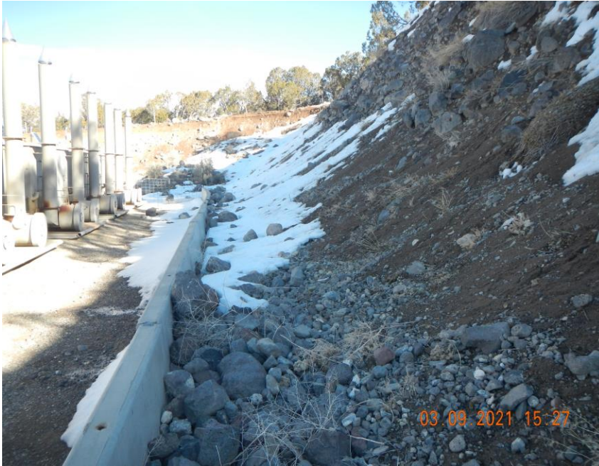
Slope not stabilized on the South cut slope
