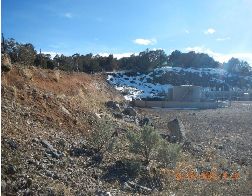
Slope not stabilized on the East cut slope
