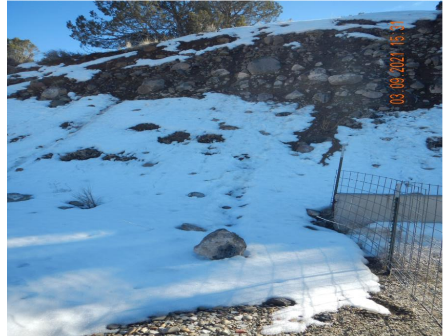
Large Rocks are falling off of cut slope onto the pad.
