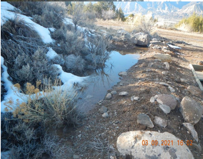
Storm Water is impounded, and saturating the soil along the pad edge and lease road used to access facility # 268858
