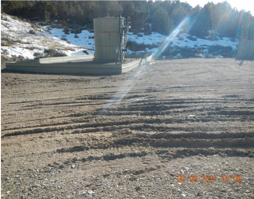
Location shows inconsistent stabilization
