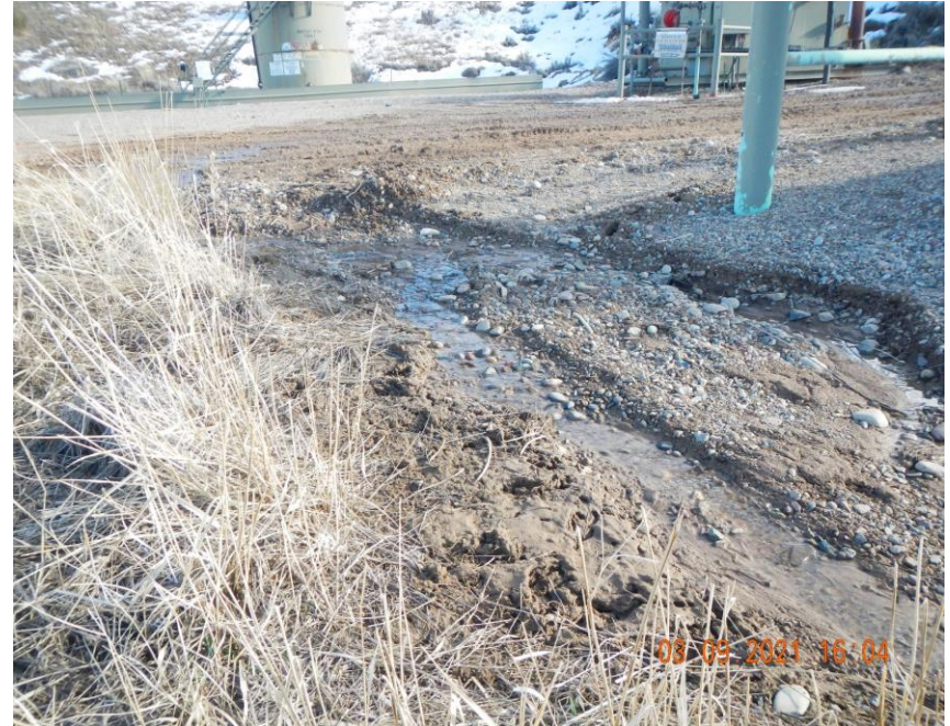
Storm water run off is causing migration of sediment from the pad surface to the vegetated areas on the North side of location.
