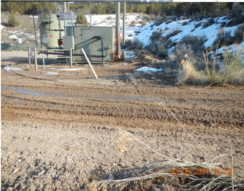
Storm water is allowed to move across location and lease road at the west side of location.
