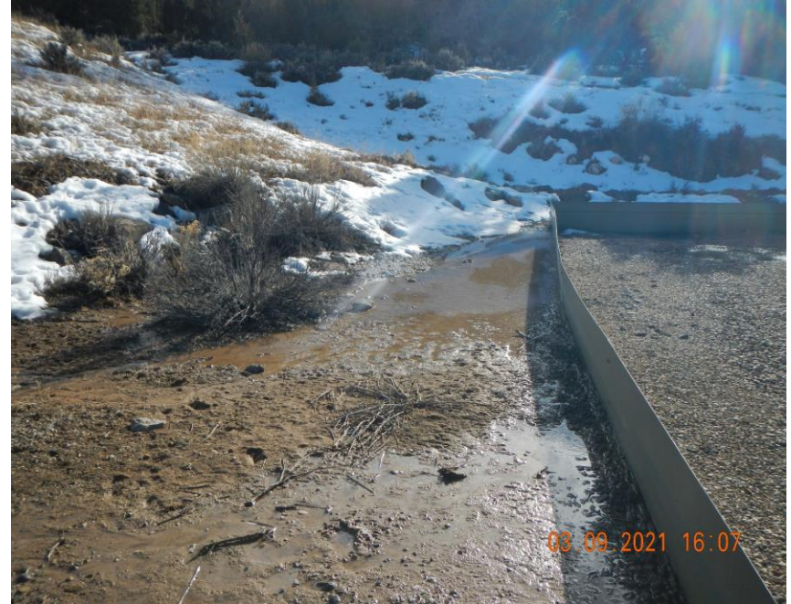
SW run-on and sediment are impeded by the production tank battery berm at the south corner of location
