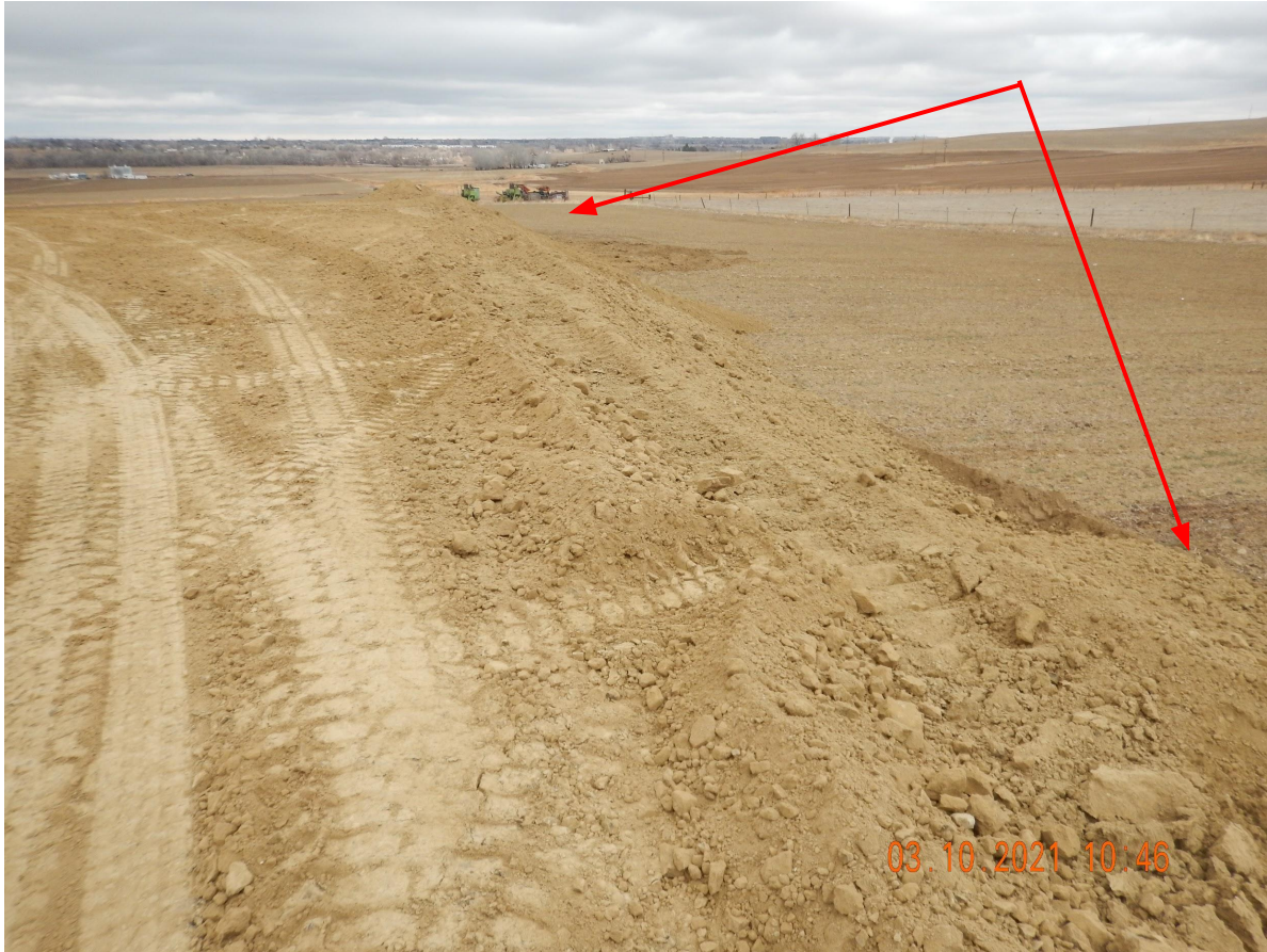
Photo 2. Photo taken from the northeastern perimeter of location, facing North. Photo illustrates there is no perimeter stormwater BMP in place during construction operations.
