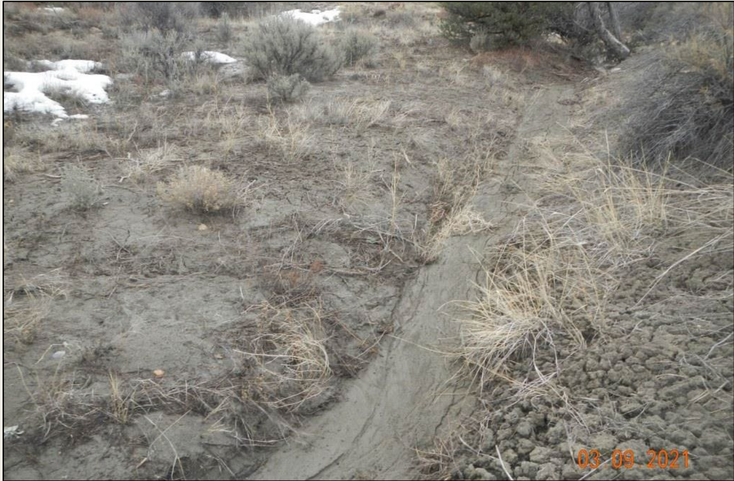
Photo 4. View of erosional channel in diversion that runs adjacent to the southern project area. Additional stabilization measures are needed here, such as channel lining.
