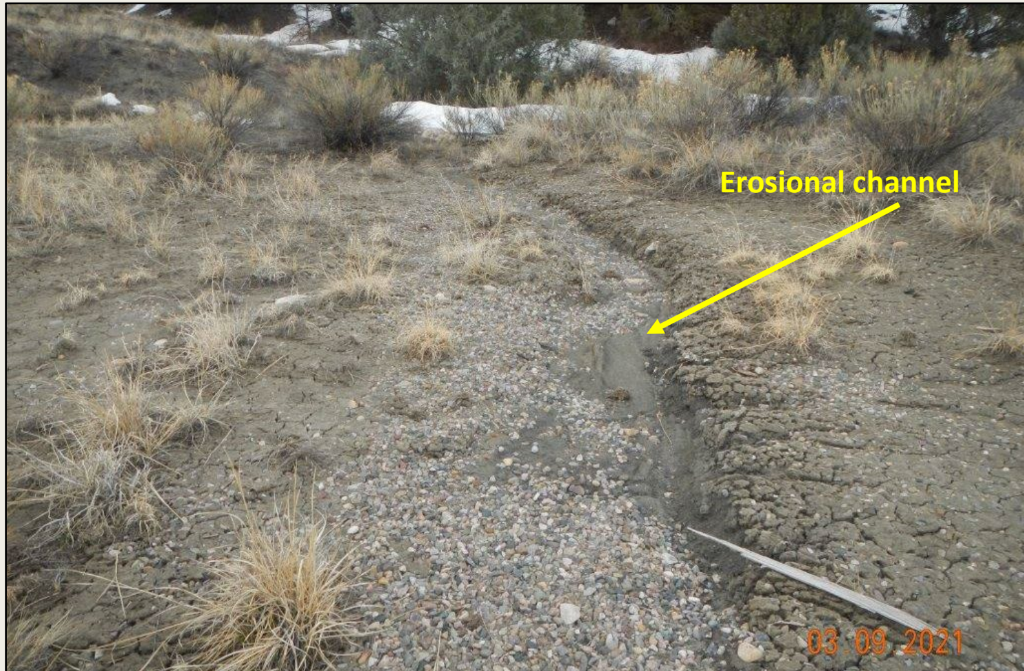
Photos 3. View of erosional channel in the southern project area, approximately 18 inches wide and 10 inches deep. Gravel placed in area is not adequate BMP.
