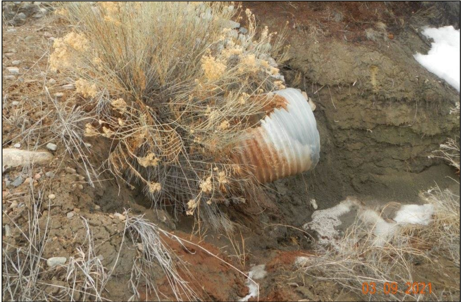
Photo 5. View of culvert outlet along the access road. Stabilization is needed around the culvert and where outflows are resulting in head-cutting from the culvert.
