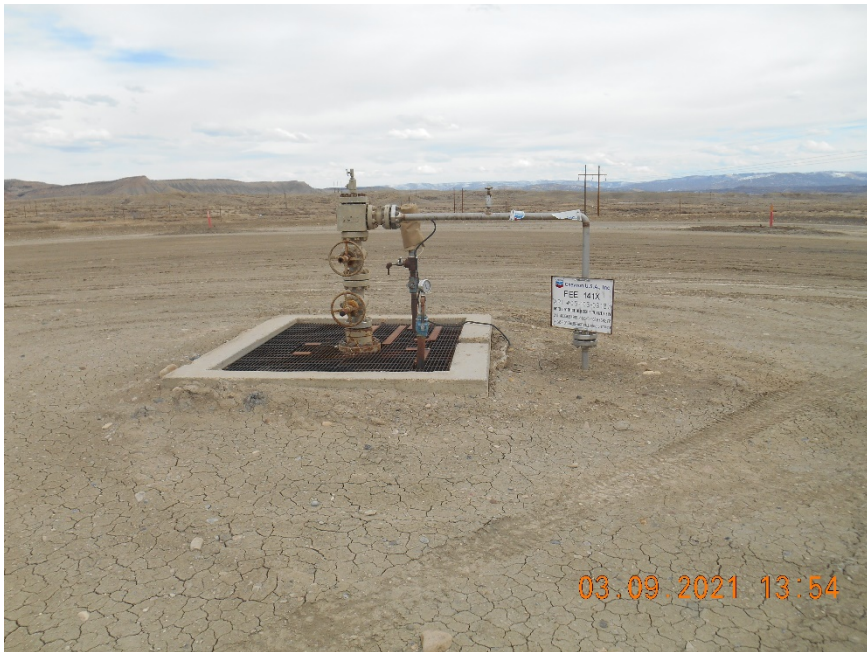
Injection wellhead.
