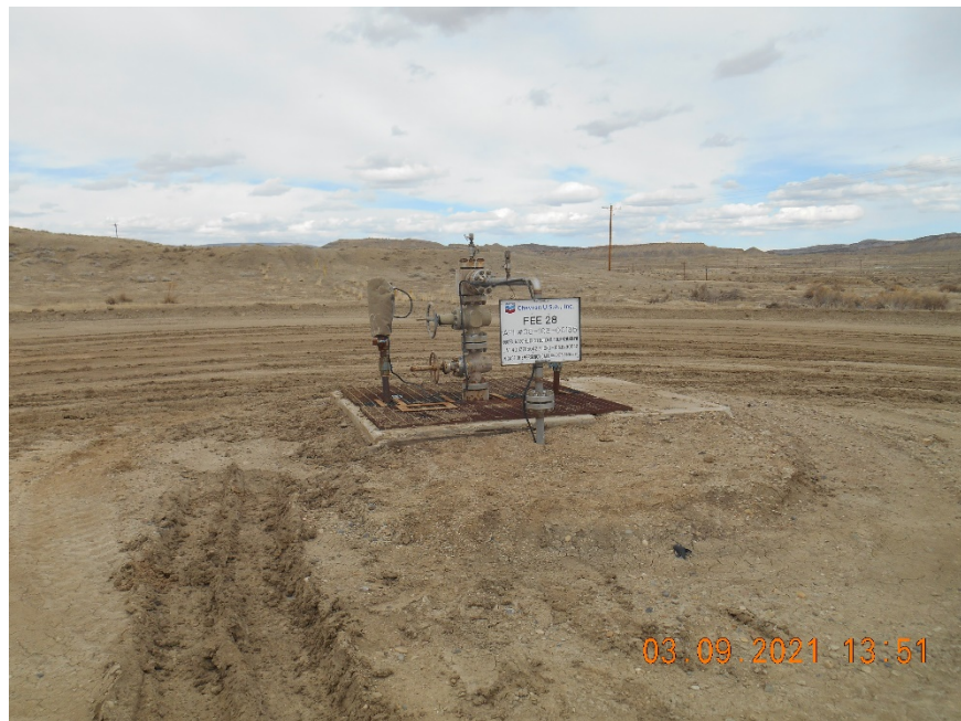
Injection wellhead.
