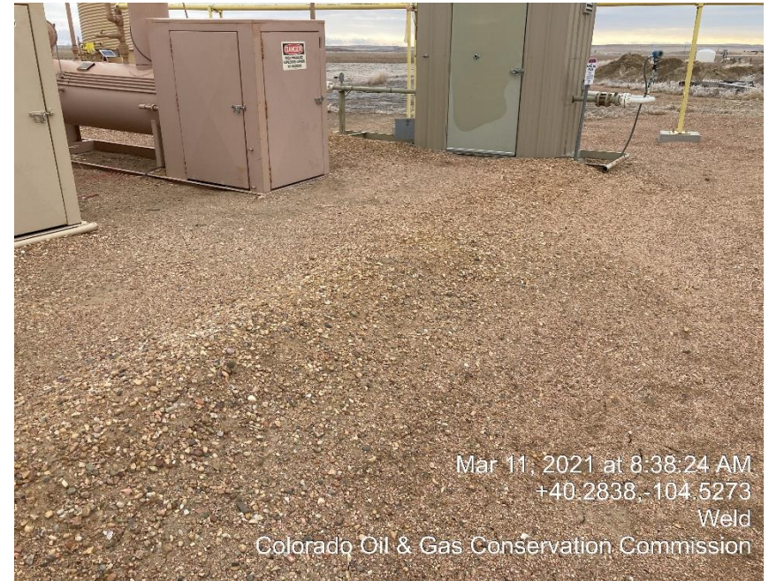
Photo #4 Weathered Berm
