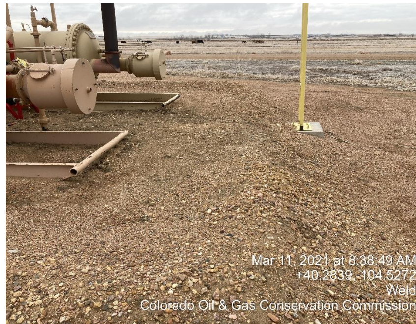
Photo #6 Weathered Berm
