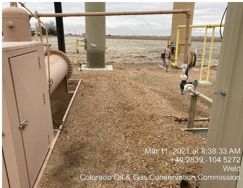
Photo #5 Weathered Berm
