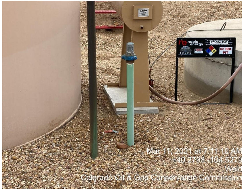
Photo #3 Unmarked Riser
