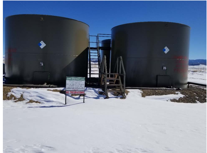
Photo 3. Battery sign and tank labels incomplete.
