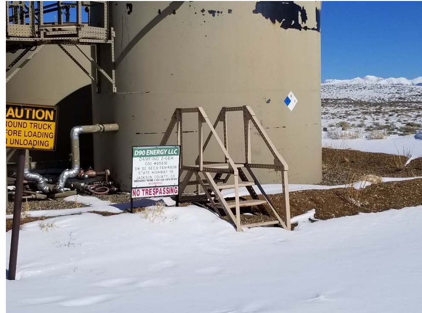
Photo 5. Battery sign and tank labels incomplete.
