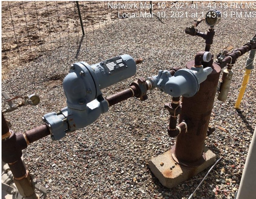
Photo #3112 In line Big and little Joe regulators
