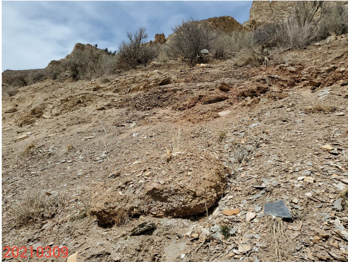
Photo 3: Photo taken from the interim areas on the north end of the Location. Photo shows that control measures to stabilize and protect the slopes are missing or insufficient. Uniform vegetative establishment on interim areas is not progressing towards 1003 standards.
