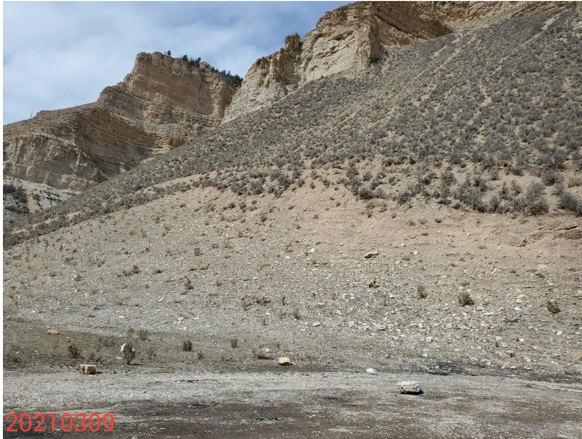
Photo 1: Photo taken from the north end of the Location, facing northwest. Photo shows interim areas where control measures to stabilize the slopes and ditch are missing or insufficient. Photo also show reclamation in these areas are not progressing towards 1003 reclamation standards.
