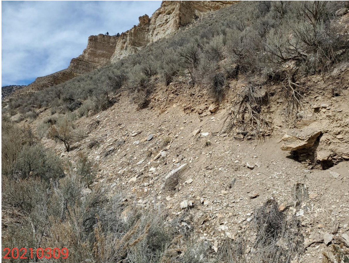
Photo 6: Photo taken from the stormwater ditch along the northern interim areas, facing west. Photo shows BMP is not in proper functioning condition; slopes along ditch have not been sufficiently stabilized; erosion degradation evident.
