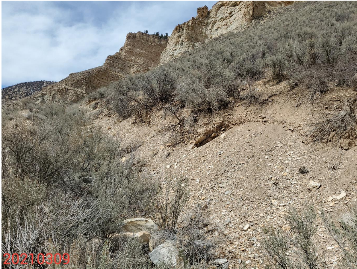
Photo 5: Photo taken from the stormwater ditch along the northern interim areas, facing west. Photo shows BMP is not in proper functioning condition; slopes along ditch have not been sufficiently stabilized; erosion degradation evident.
