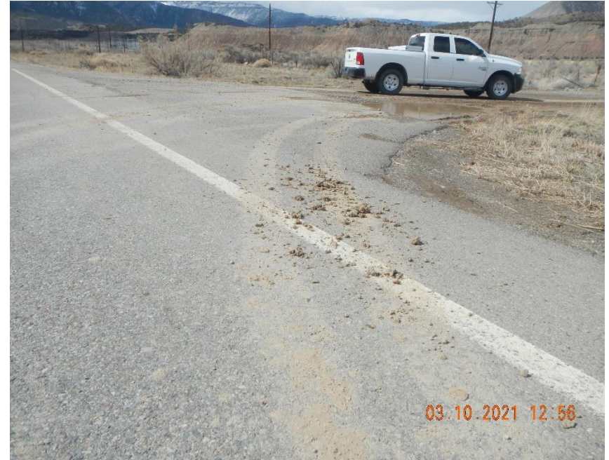
Tracking sediment on to Hwy 6.
