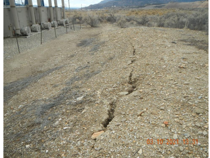
Settling crack on diversion berm behind tank battery.
