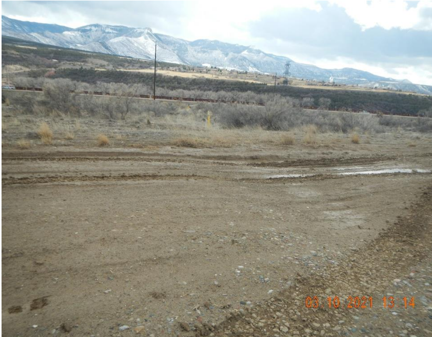
Low water drain across access road needs maintained. Coordinates 39.47173 108.02898
