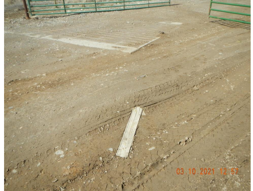
Marker ran over and partial broken at ground on expand entrance.
