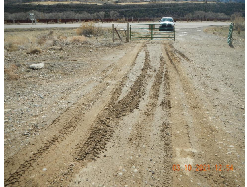
Expanded road not stable and no BMPs in place.
