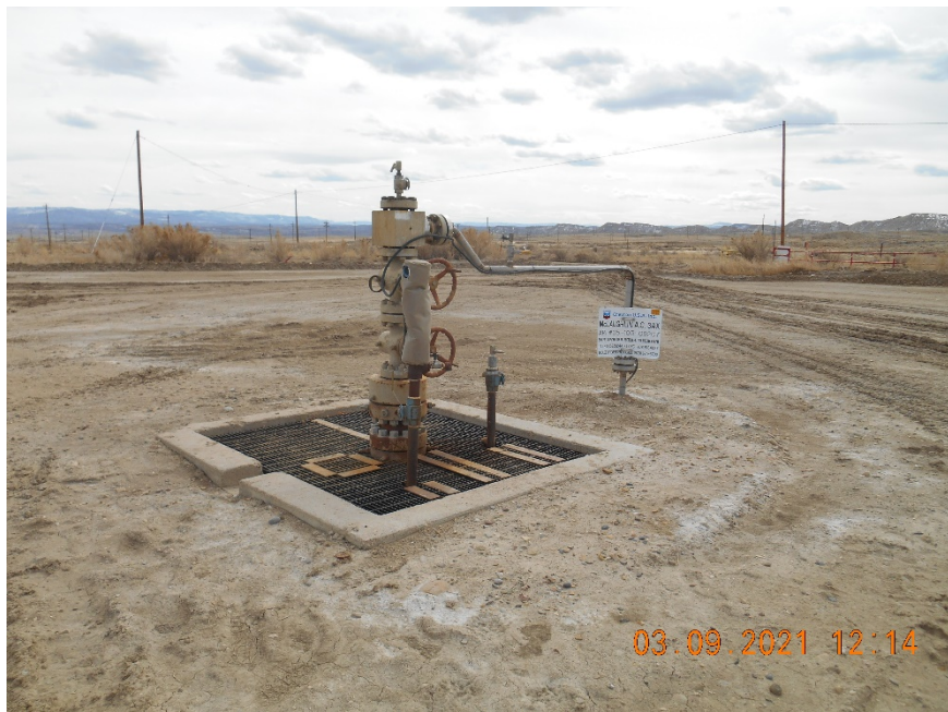
Injection wellhead
