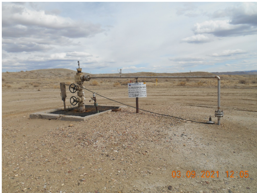
Injection wellhead
