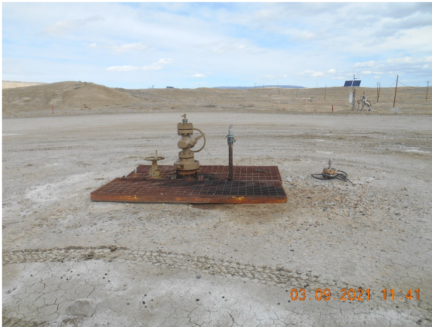
Injection wellhead- Temporarily Abandoned
