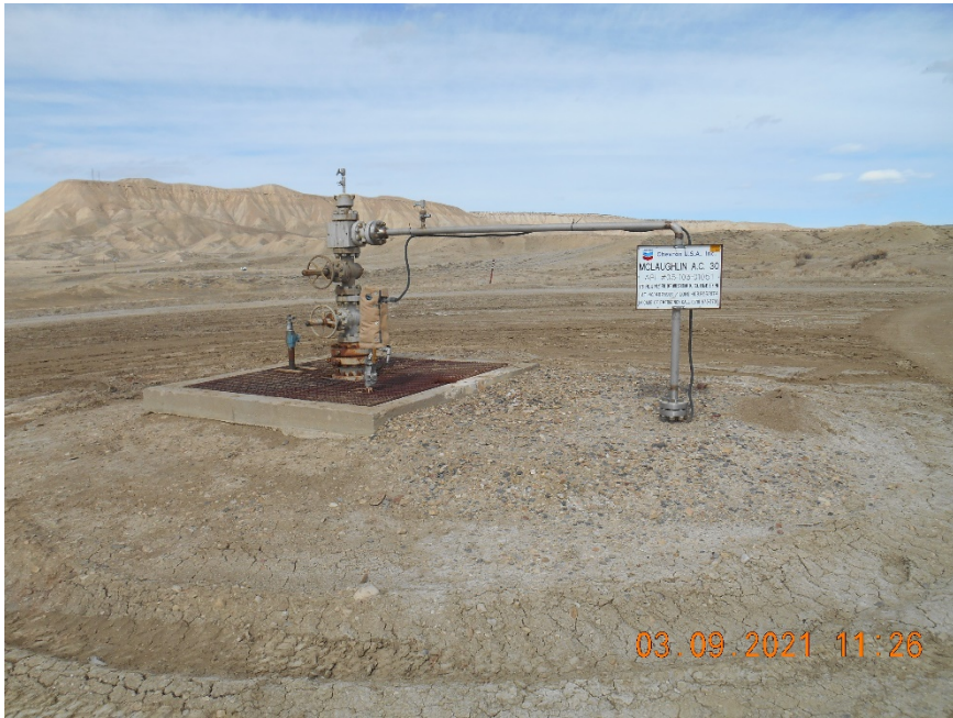
Injection wellhead
