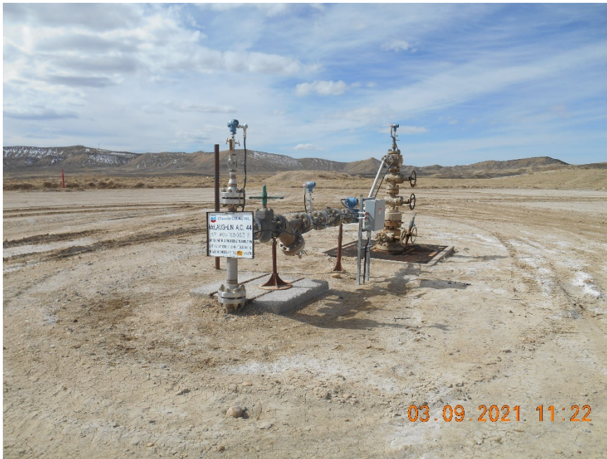
SWD Injection wellhead
