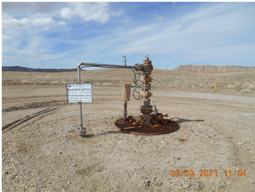
Injection wellhead
