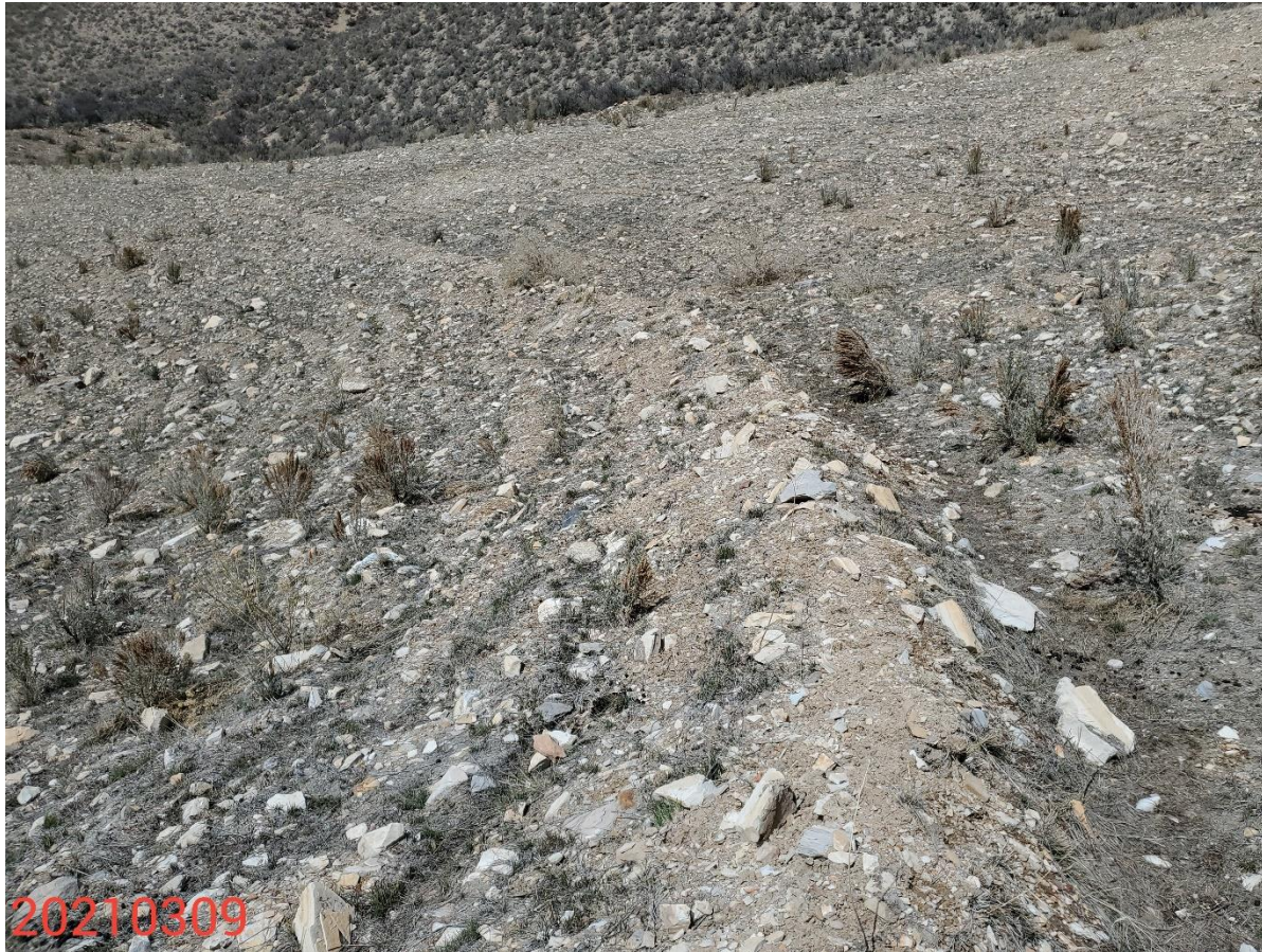
Photo 7: Photo taken from the northeastern interim areas. Interim areas appear to be progressing towards COGCC 1003 Standards. Photo also shows stormwater run-on ditch and berm installed at interim areas.
