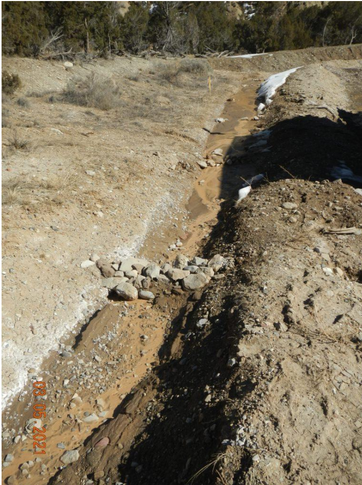
Photo#13: BMPs needing repair/maintenance.
