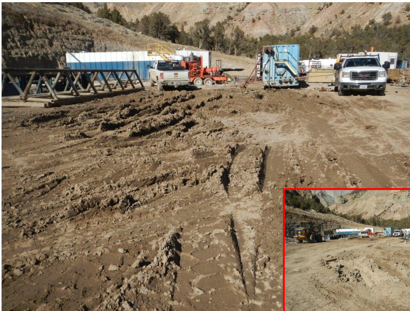
Photo#10: Rutting on portions of pad.
