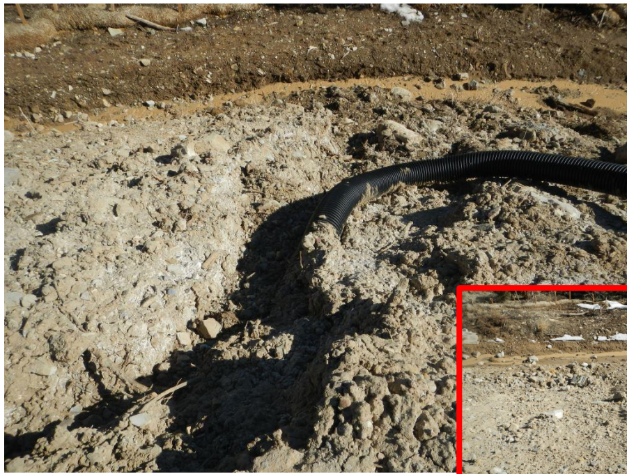
Photo#6: Erosion, degradation of Fill slopes.
