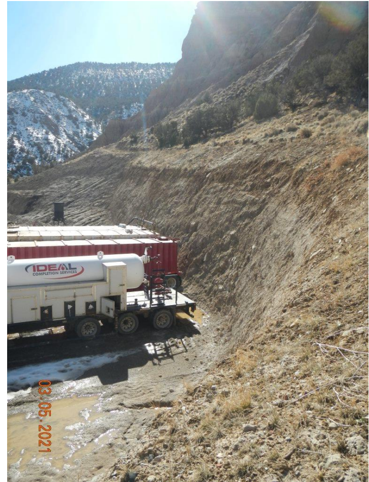
Photo#5: Sediment migration & erosion on Cut slope.
