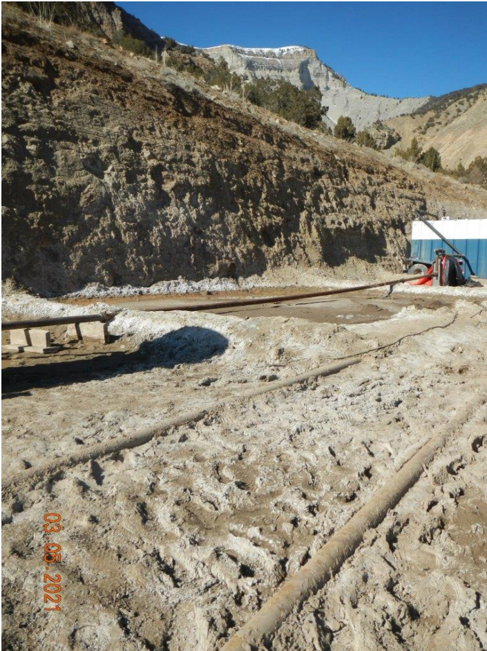
Photo#4: Sediment migration & erosion on Cut slope.
