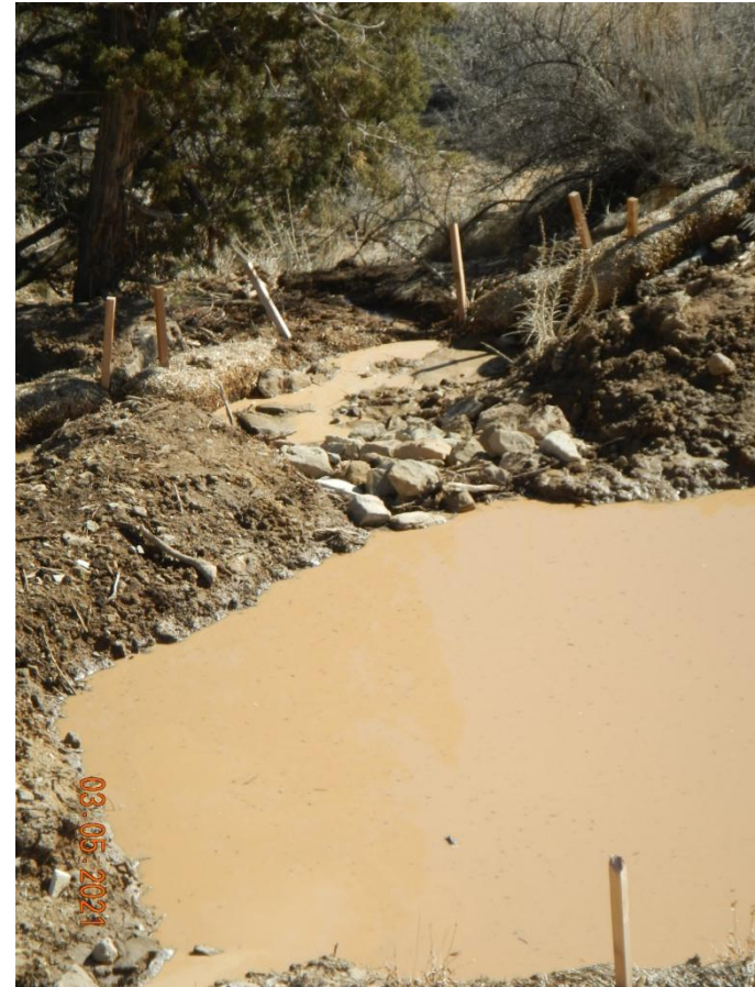
Photo#12: BMPs needing repair/maintenance
