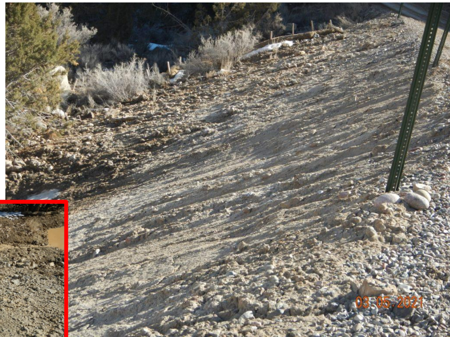
Photo#7: Erosion, degradation of Fill slopes.
