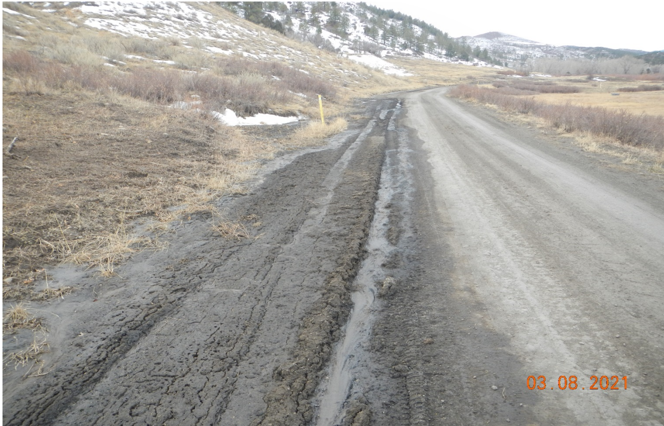
Photo 3. The side of the road is filled in with sediment which is preventing stormwater from draining to the culvert.
