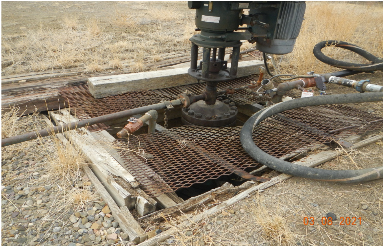
Photo 7. There is opening where the still grate is around the wellhead. This area needs to be covered to prevent wildlife entry.
