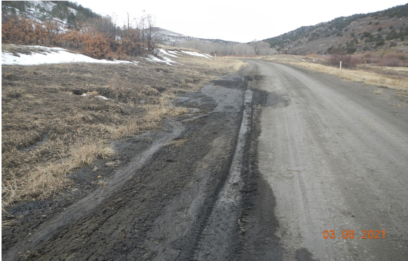
Photo 4. Sediment is accumulating along the main road.
