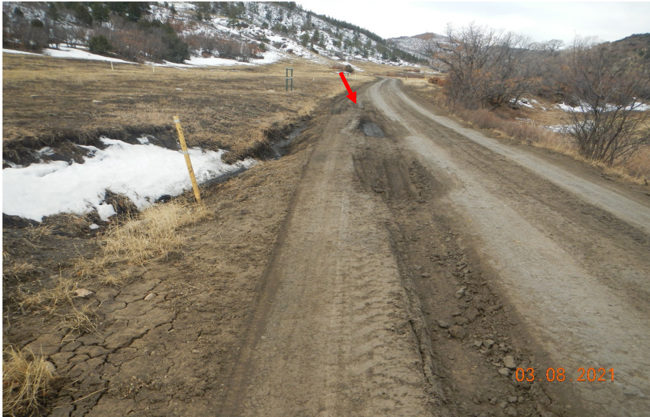
Photo 2. Stormwater is not properly diverted at the red arrow causing stormwater to pool in the vehicle ruts. This area needs to be repaired. (Lat/Long:37.071679,-104.91145) Previous corrective action was not performed.
