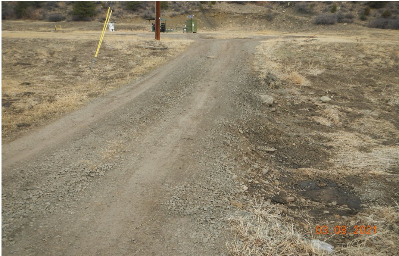
Photo 5. Water from the river caused erosion across the access road.
