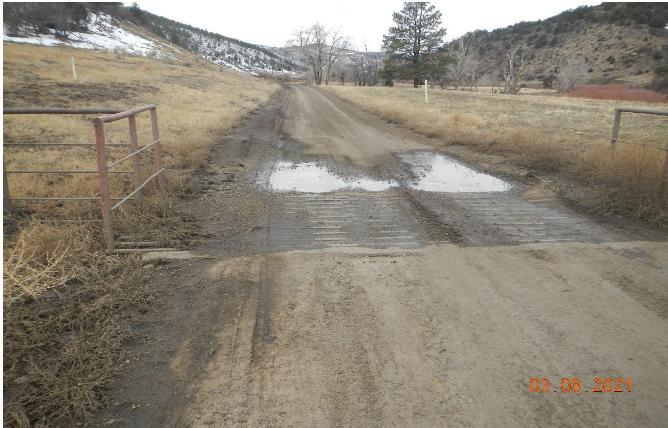
Photo 1. The cattle guard along the main road near the Bingham campground is filled in with sediment. The cattle guard needs to be cleaned out and maintained. Previous corrective action was not performed.
