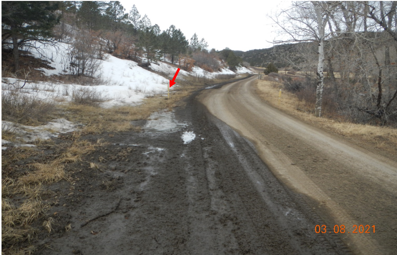
Photo 2. The culvert shown at red arrow is filled in with sediment. Stormwater is not directed toward the culvert and is flowing down the road. Lat/Long:37.06585,-104.93198.
