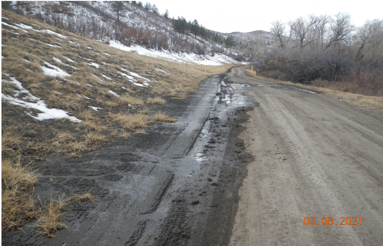
Photo 1. There is sediment deposition onto the main road. Stormwater is not properly diverted.
