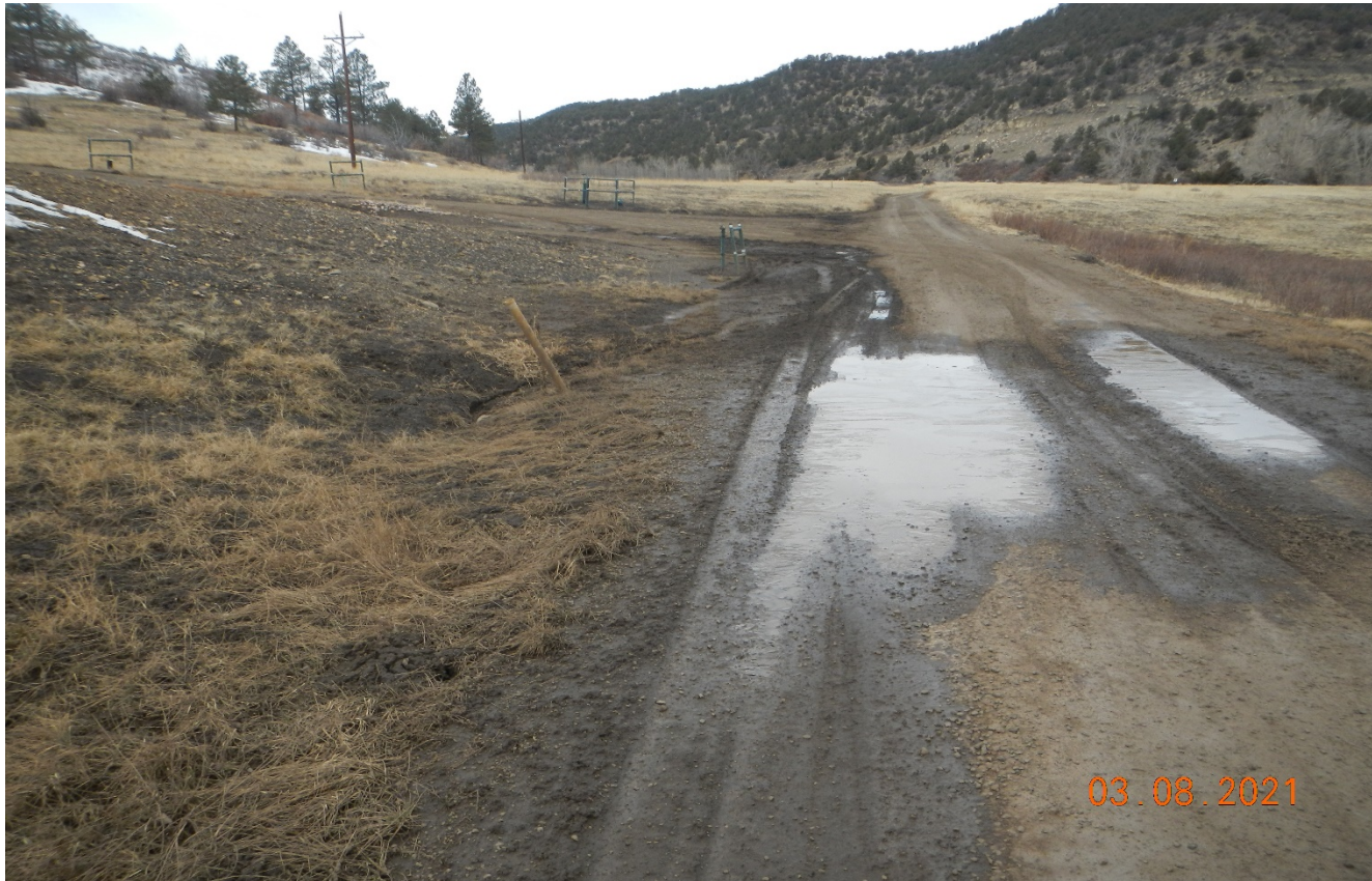
Photo 3. Facing west along main road near the location. Stormwater is not directed toward the culvert and is pooling on the road.
