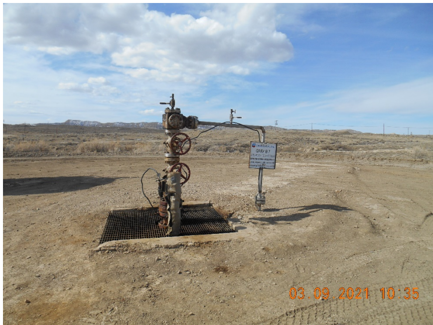
Injection wellhead
