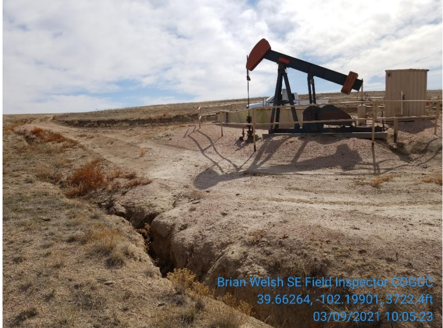
2. Erosion on access
