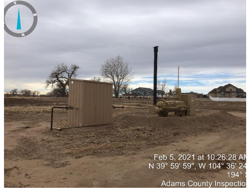
Photo #2 Meter & Separator.
