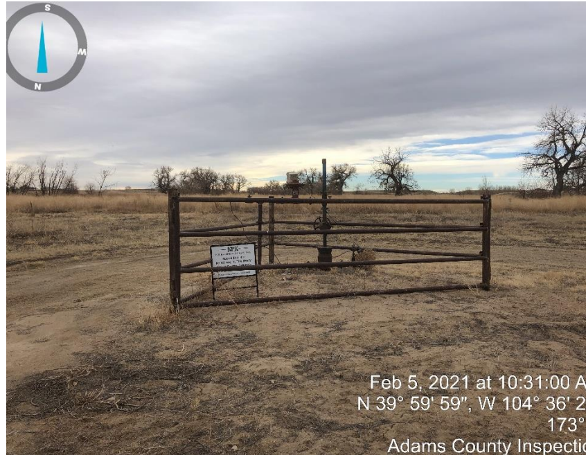
Photo #3 Well Head.
