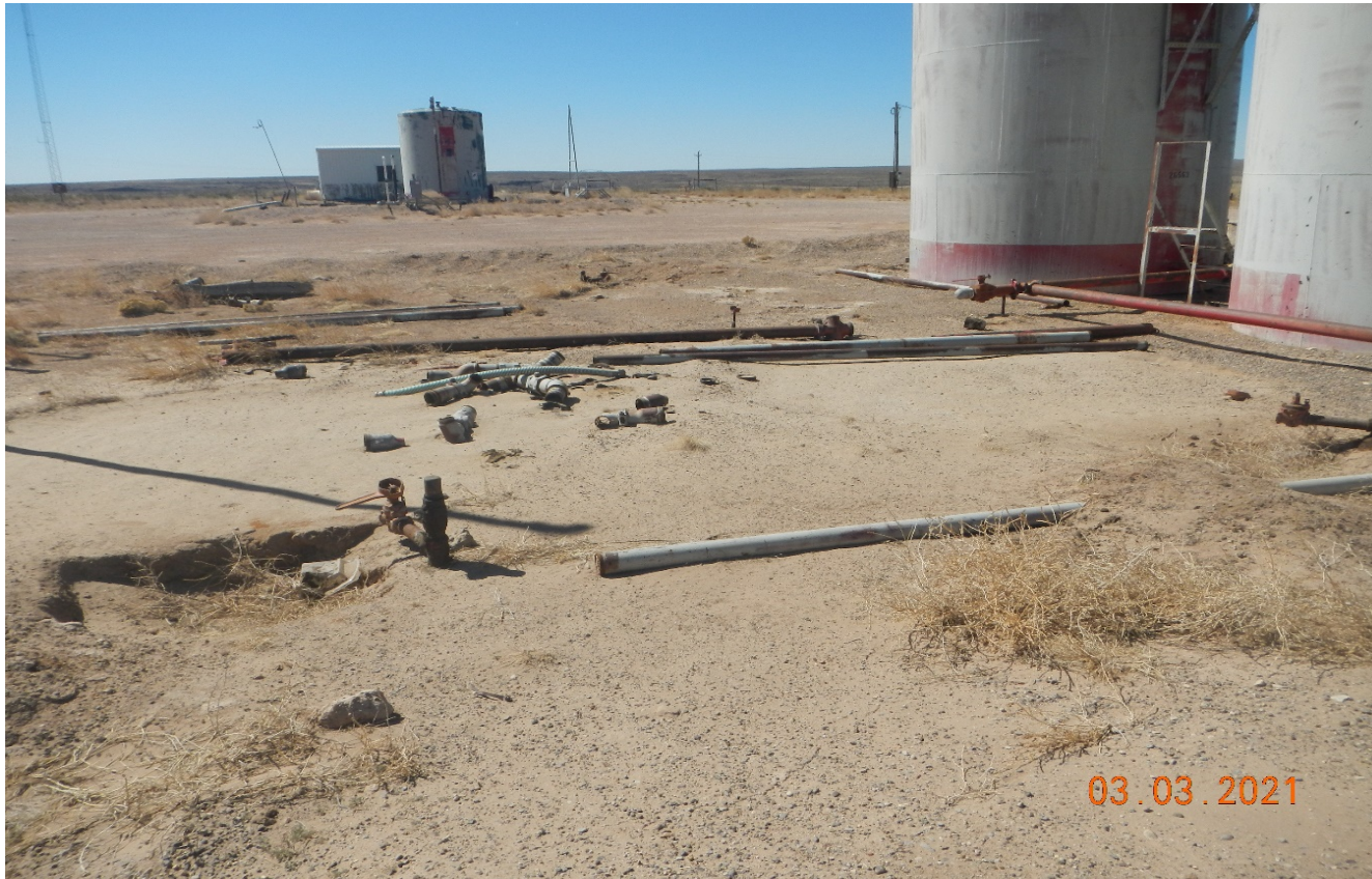
Photo 5. It appears a tank has been removed. All equipment and pipe risers need to be removed.
