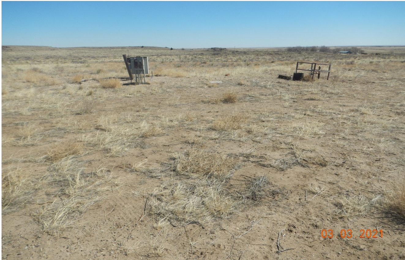
Photo 2. There is a pipe riser and electric utility that remains at the east side of the location. All equipment should have been removed within 3 months of abandoning the well.
