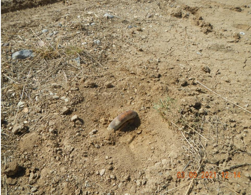
Unmarked deadman south east corner of location along roadway.
