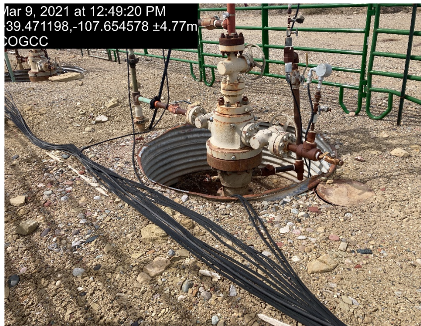
Well head cellar rings with out any way for wildlife to escape
