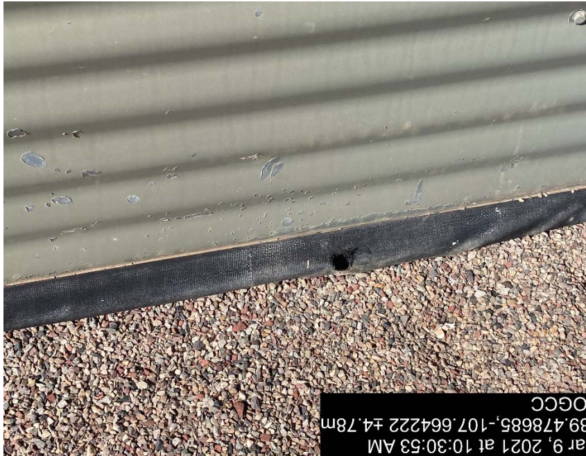
Multiple holes in tank containment liner
