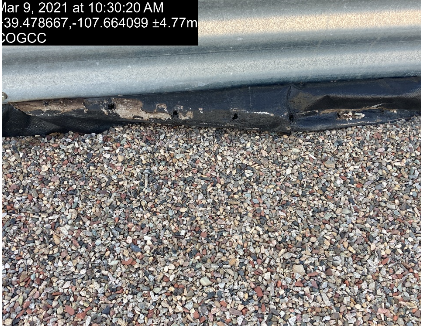
Multiple holes in tank containment liner
