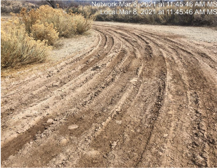
Photo #3088 3086 Rutting present on location due to lack of stabilization.
