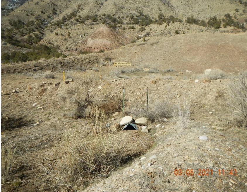
Culvert just before main road and access road intersection needs maintained.
