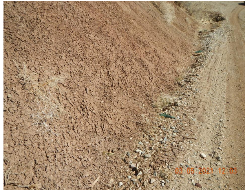
Rock sack covered by sediment.
