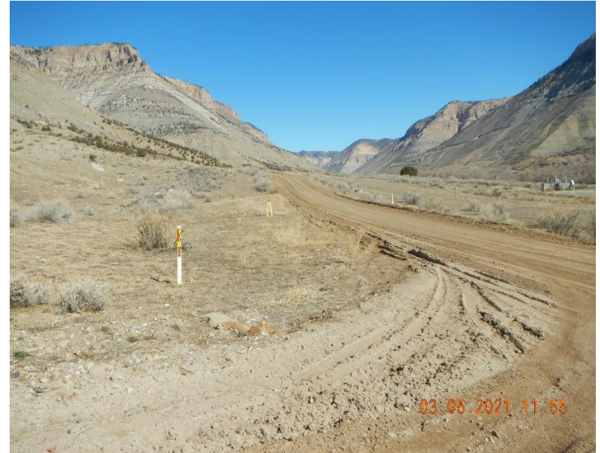
Ditch is damaged by rutting.
