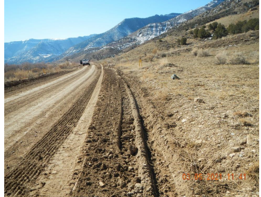
Tire ruts in roadside ditch.
