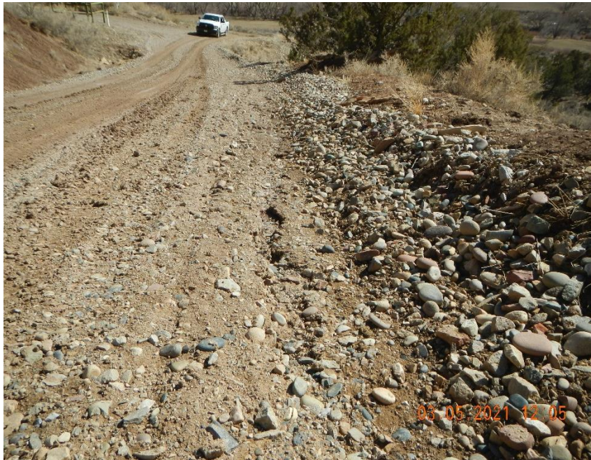
Riling erosion down road side along ditch.
