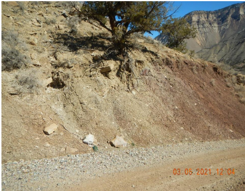
Sediment from cut wall sloughing into ditch.
