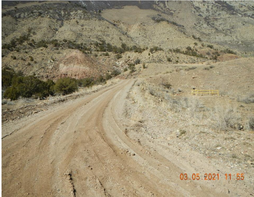
Ditch is damaged by rutting.
