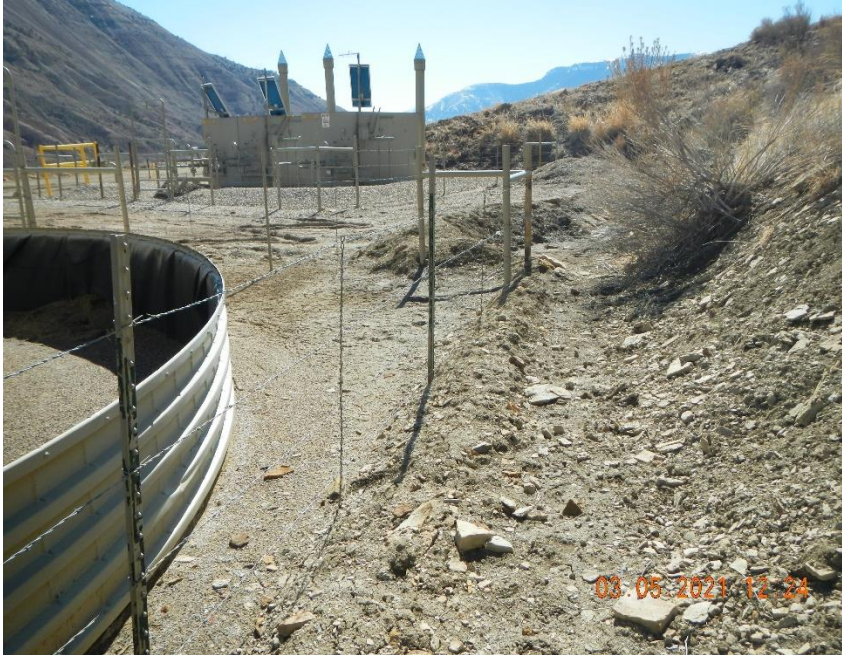
Sediment build up behind tank battery.
