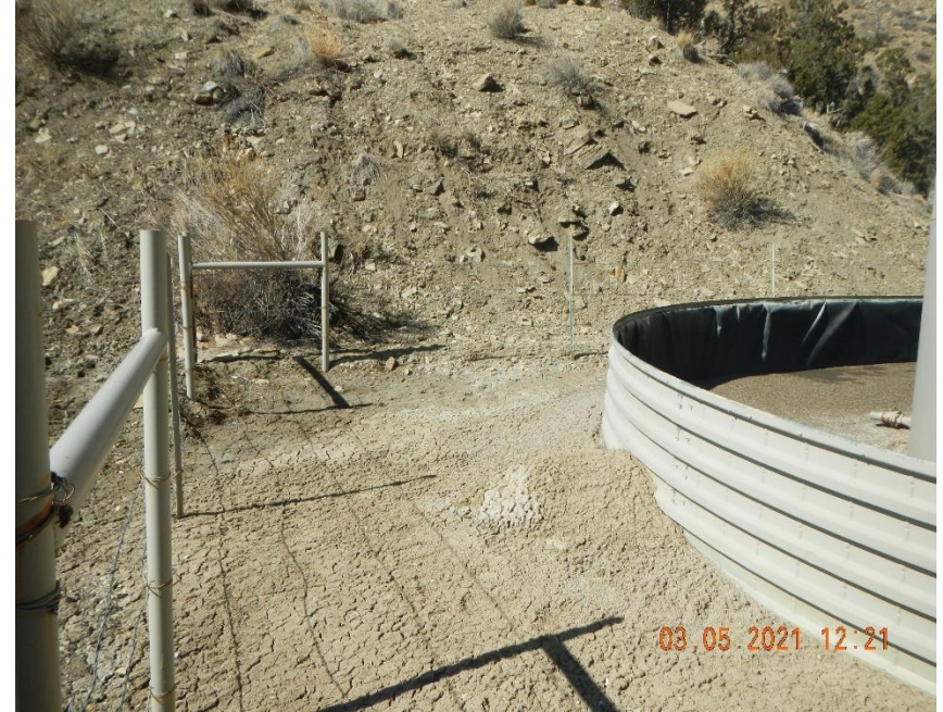
Sediment build up at tank berm.
