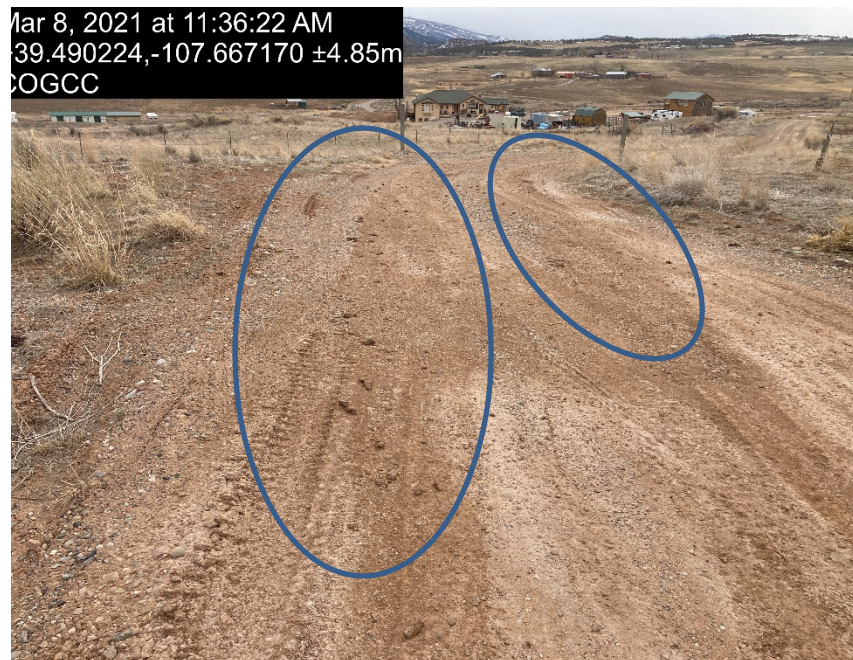
Evidence of lack of tracking controls
