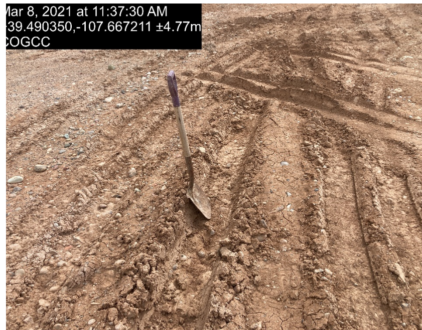
Lack of stabilization/compaction
