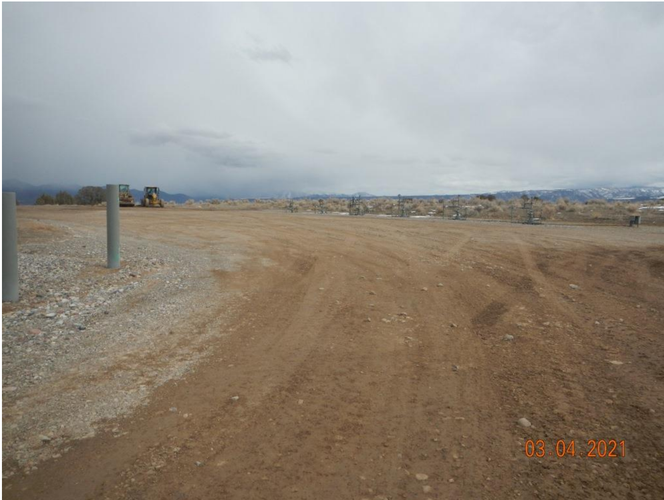
Photo#1: Overview of Location from entry.
