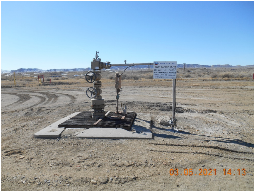
Injection wellhead
