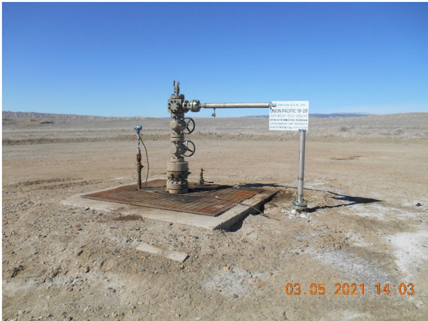
Injection wellhead
